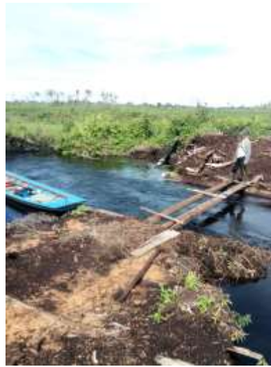
After Repairment by PT Limpah (photo taken 16/12/19)
